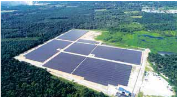
First LSS Project COD in LSS2 Scheme - 12.5MWp Kamunting Ground Mounted Large Scale Solar Farm
