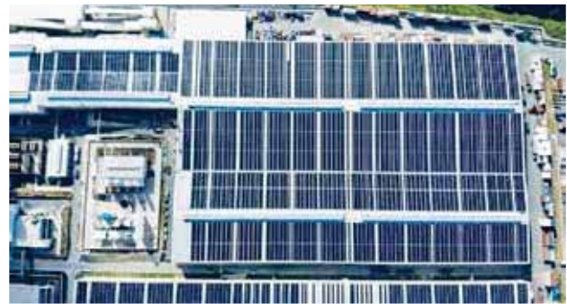
7.7MWp Rooftop Solar Project Complete Installation within 40 days
