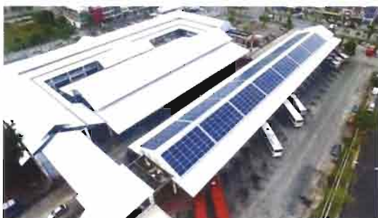
Rooftop - Retrofit installation
