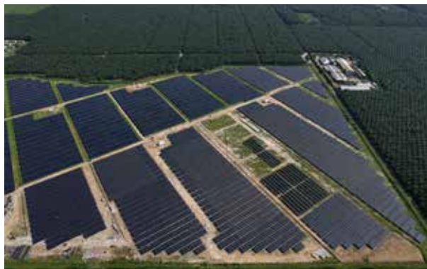
Manjung, Perak ~17.2MWp COD date: Dec-23
