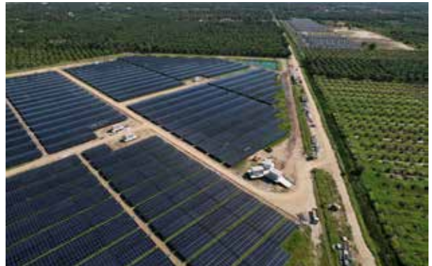
Kuala Selangor, Selangor ~20.5MWp COD date: Nov-23
