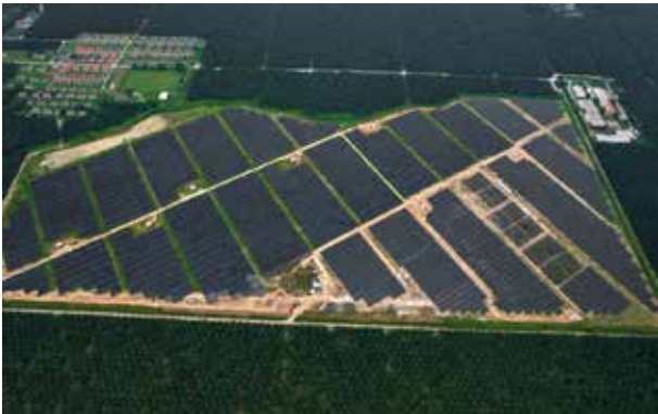
Manjung, Perak ~29.6MWp COD date: Aug-23
